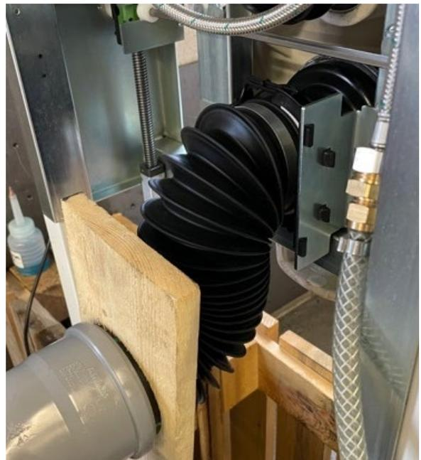
**e.** Cut threaded rods to length and secure them in the frame
