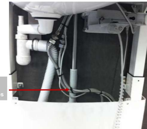
Recommended fixation of the hoses and wires
