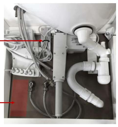
Recommended placement of electrical installation
